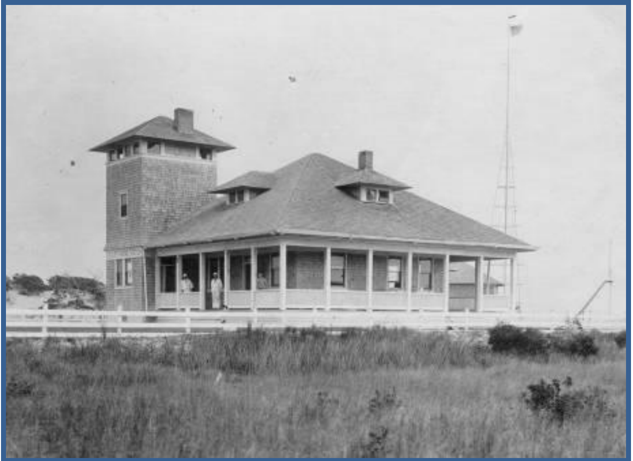
The Original Bogue Inlet Lifesaving Station
